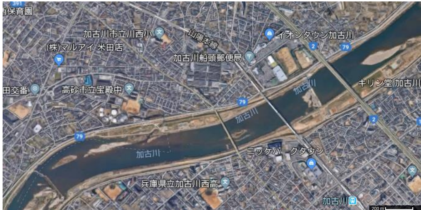
Satellite photo downstream of the Kakogawa River
